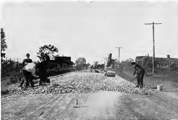
Spreading and binding foundation stone.
